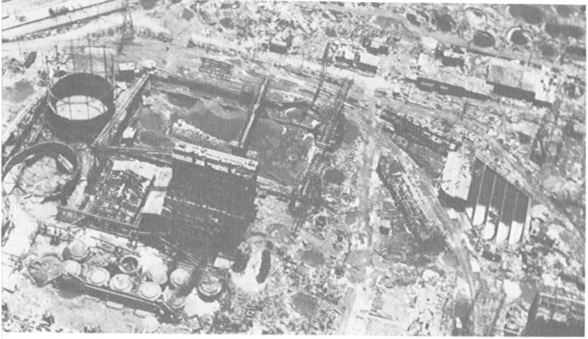
THIS OIL REFINERY IN THE TOKYO AREA was a key target during the final five months of the war against Japan.
